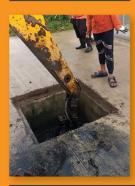
Once the clamshell bucket is in the manhole. We can spread the clamshell bucket to fill the manhole area. Then lower the clamshell bucket until reach to the debris, then gorge the clamshell bucket mouth to bring the debris out of the manhole.
