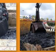
Move the clamshell bucket and discharge the debris into a truck to be disposed of properly.
