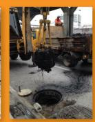
This clamshell bucket can scoop debris in the manhole at full rate at a time. It's more than manual labor to pick it up.
