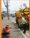
Take the PVC pipe, pass the end of the rope or sling from one end of the sewer to the other end of the sewer.
