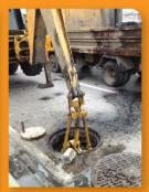
Then take the clamshell bucket attached to the JCB or small back hoe and drop it into the manhole in the shutting mouth state.
