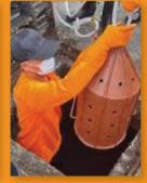
Take the end of the rope or sling about the sewer cleaning debris basket mouth, and the rope or sling is attached to the hook on the bottom for used in case of pulling back.
